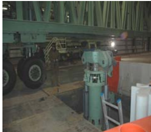
Top Portion in Pit Ready to Install
