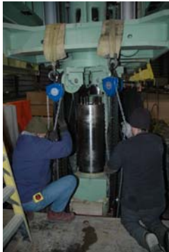
Lower Module Portion Hoisted into Position
