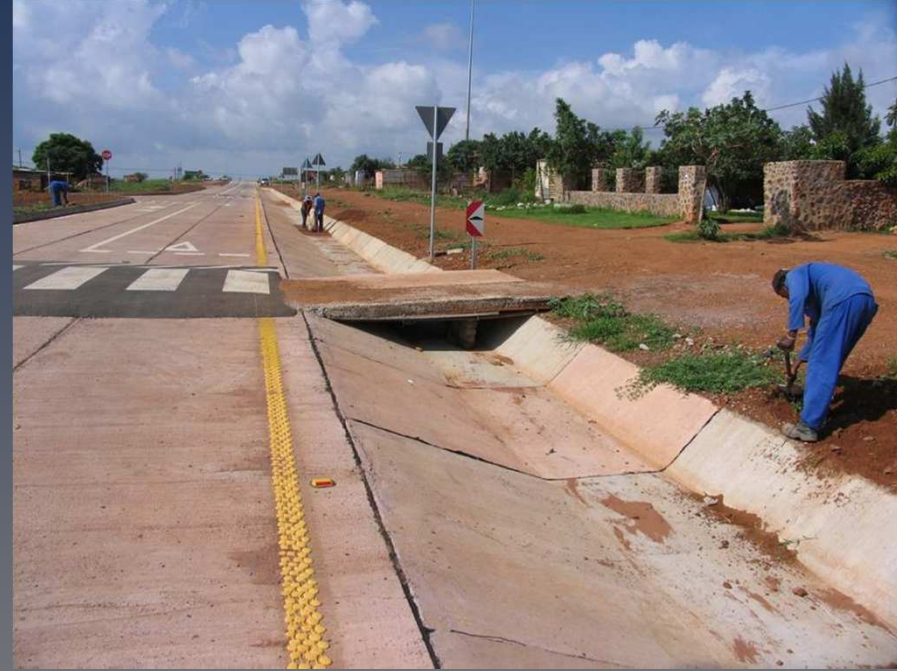
Completed UTRCP road with side drain
