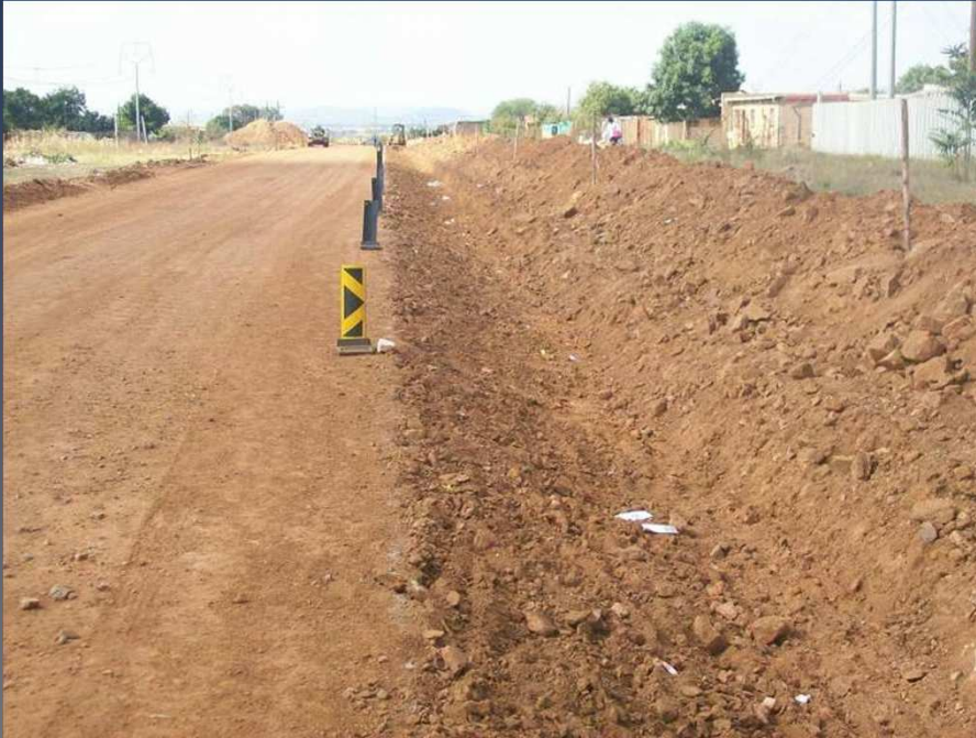
Earthworks and shaping of in-situ layer
