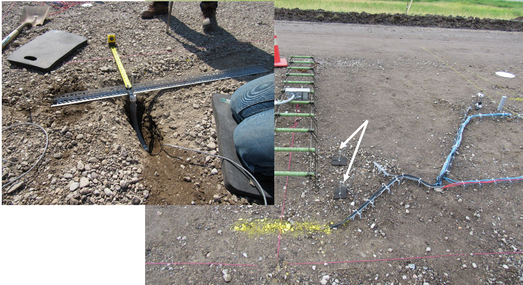
Magnetic induction slab lift sensors
