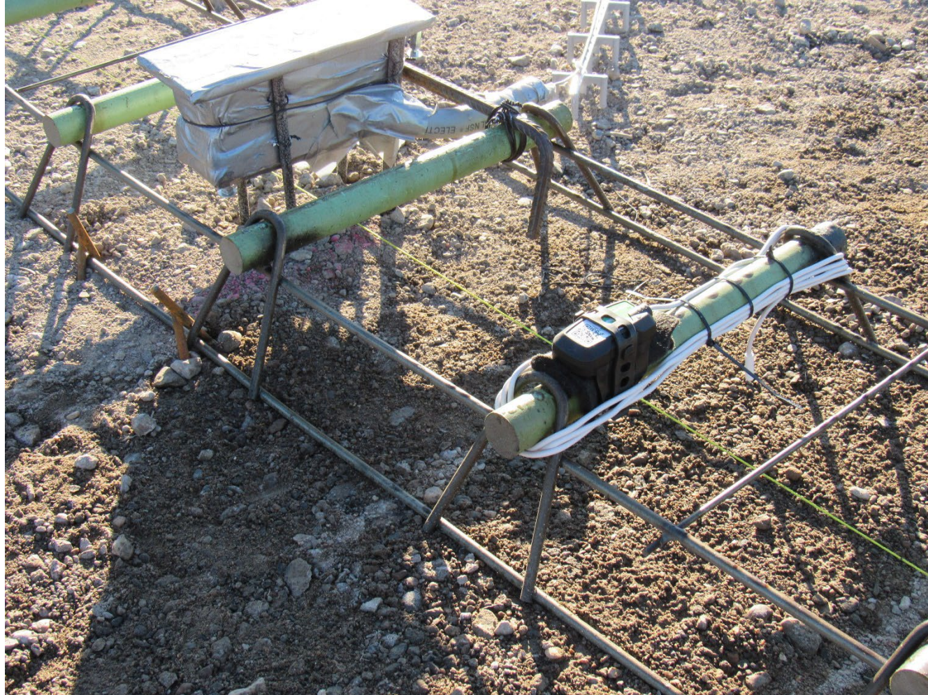
Joint opening sensor blockout and maturity sensor
