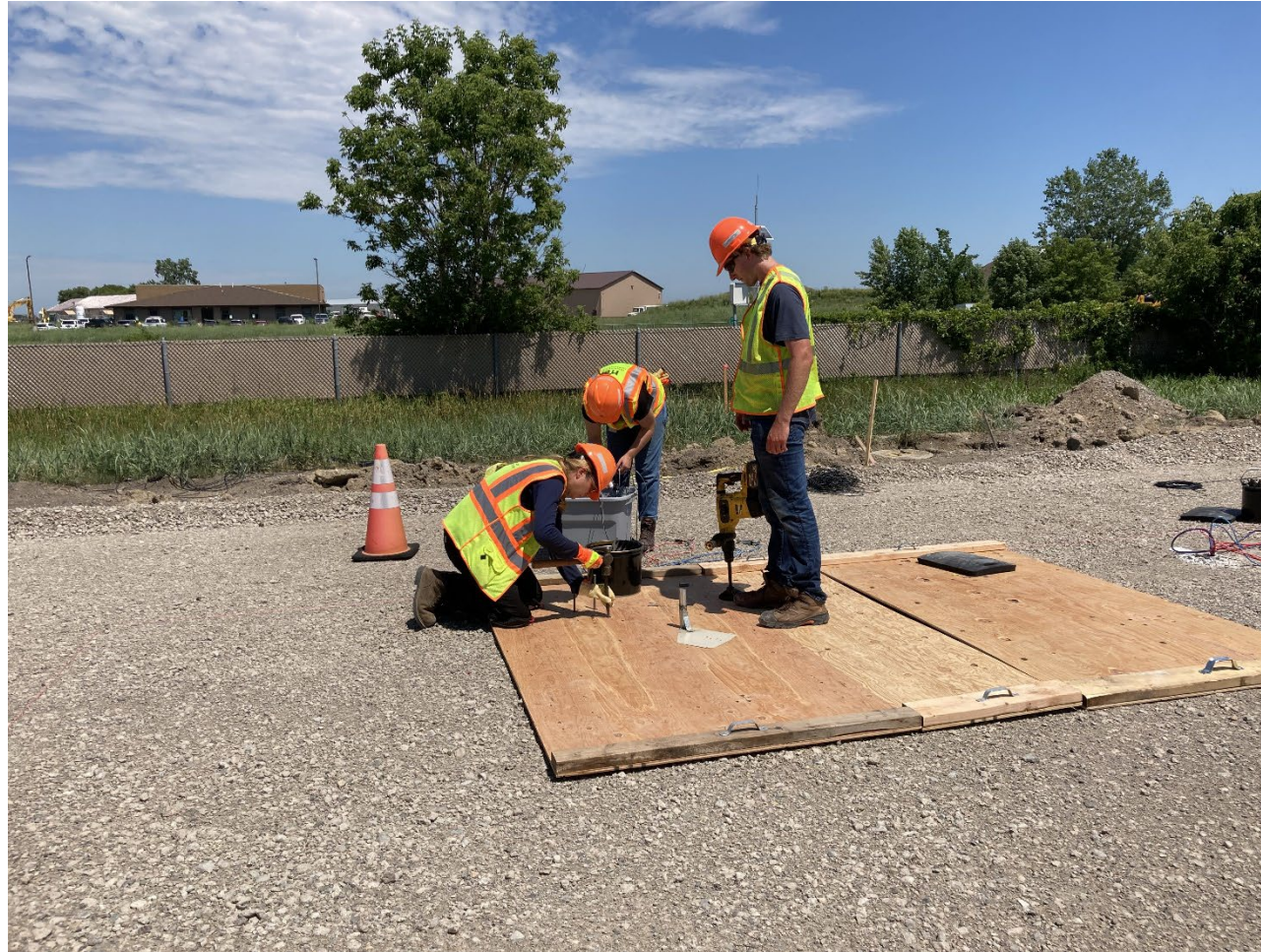
Plywood templates to locate support dowels
